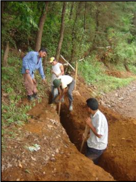
Villagers digging trenches for the conduction line
