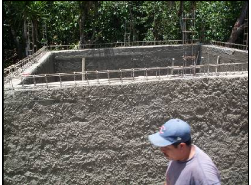
Distribution tank 75% completed
